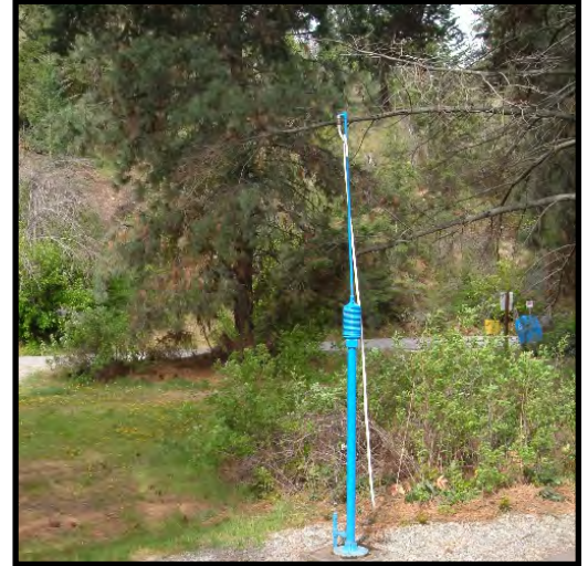
Outdoor faucet/city water source
