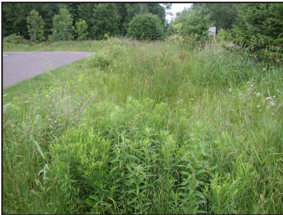
Infiltration swale with native grasses
