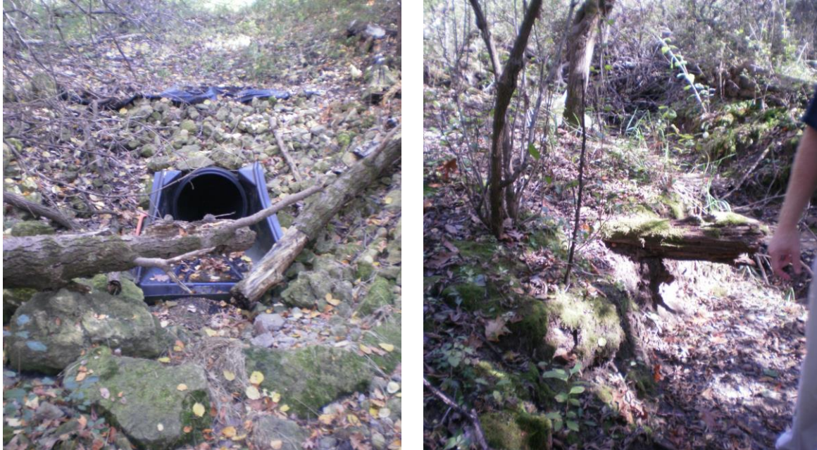
Figure 40. County Road 7 swales drainage pipe (left) and SW-2 gully (right)
