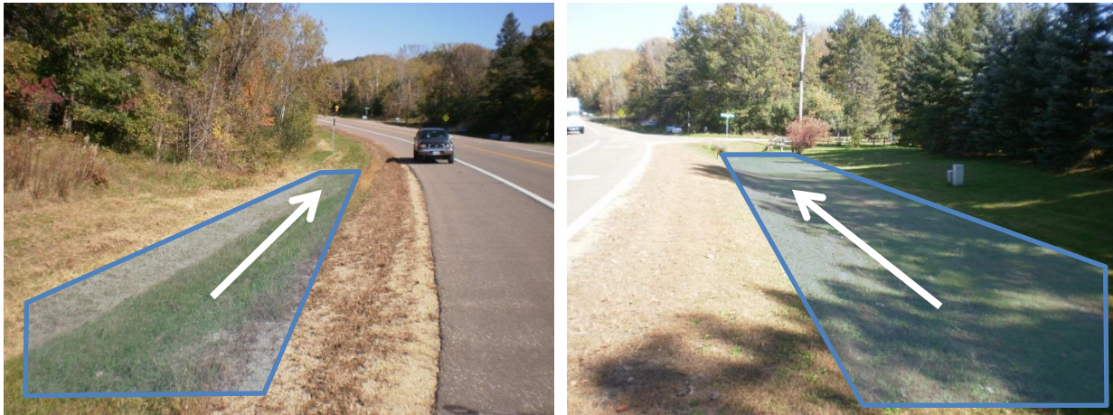
Figure 41. Potential retrofit areas of the road right of way swales discharging to the SW-2 gully. The shading denotes areas to be excavated and backfilled. The arrows show general flow direction.
